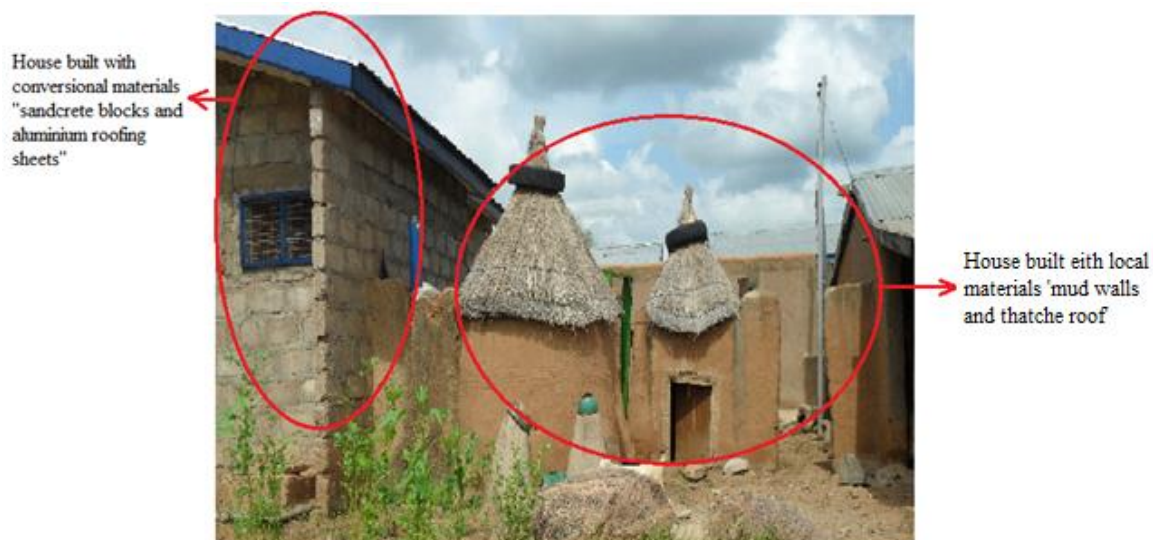
Figure 1: Houses built with local and conversional materials in Dorongo, Upper East Region
