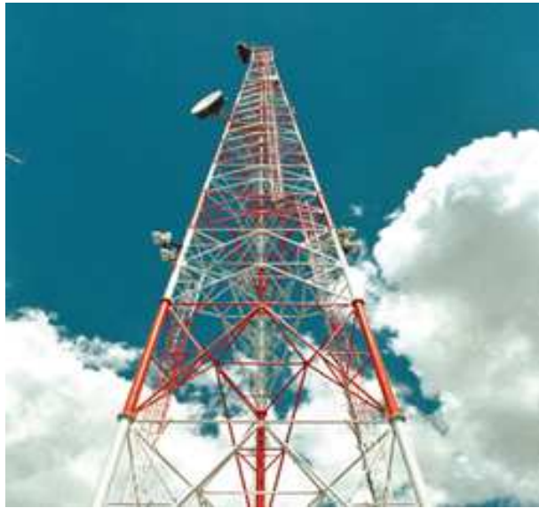
Figure 1: legged Tubular Tower
