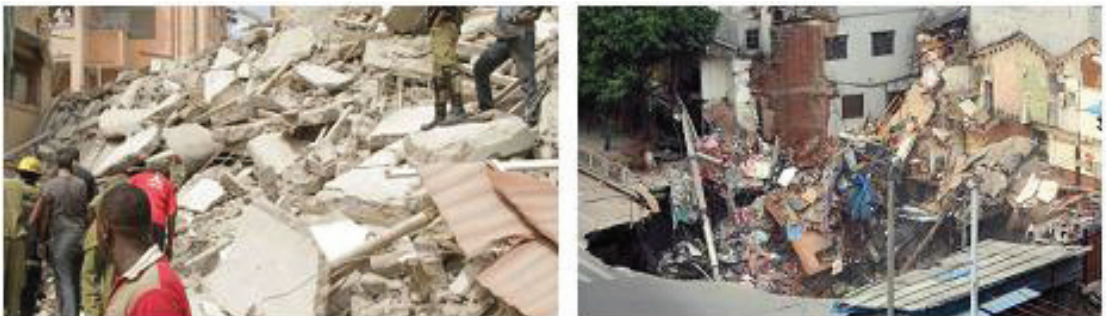
External View of Building after Collapse
