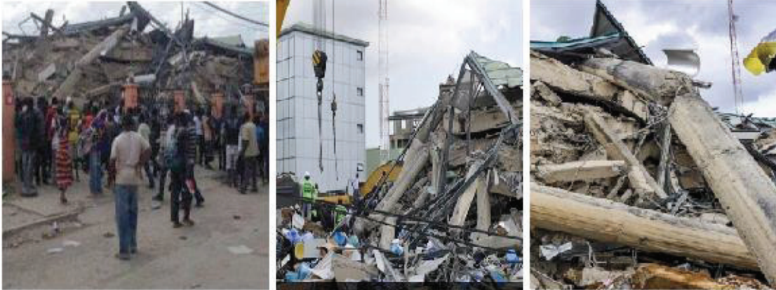
External View of Building after Collapse
