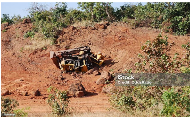
Figure 4. 6 : Quantity surveyors and excavators on construction sit
