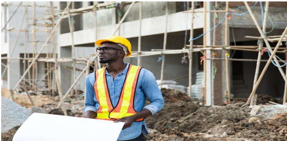
Figure 4. 5 : Photo of contractor reading building plans in protective safety hard hat looking at blueprint plans on construction site.
