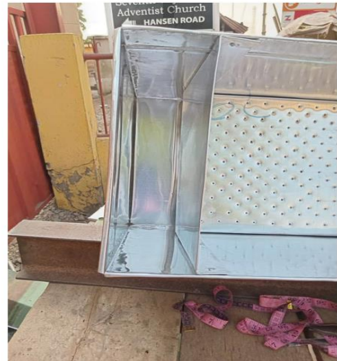
PLATE 4 Plate 4: fitting of outlet and under drain
