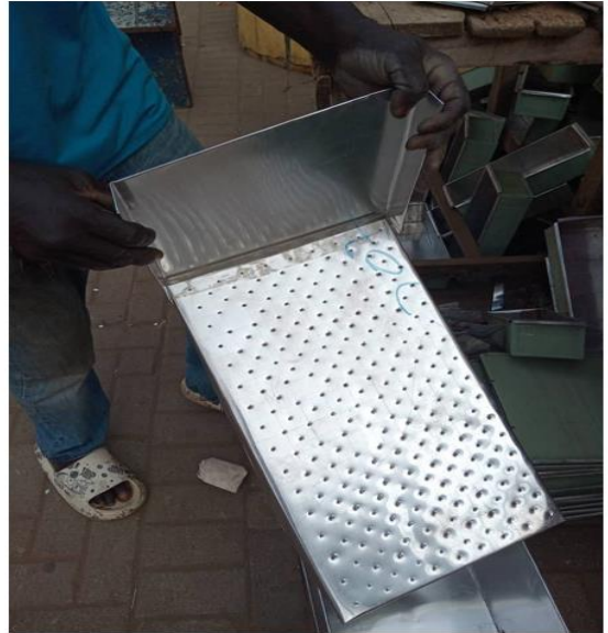
PLATE 3 Plate 2: construction of underdrain
