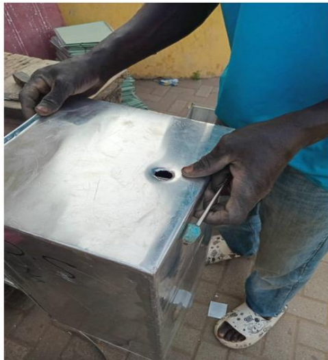
PLATE 3 Plate 3: construction of filter outlet
