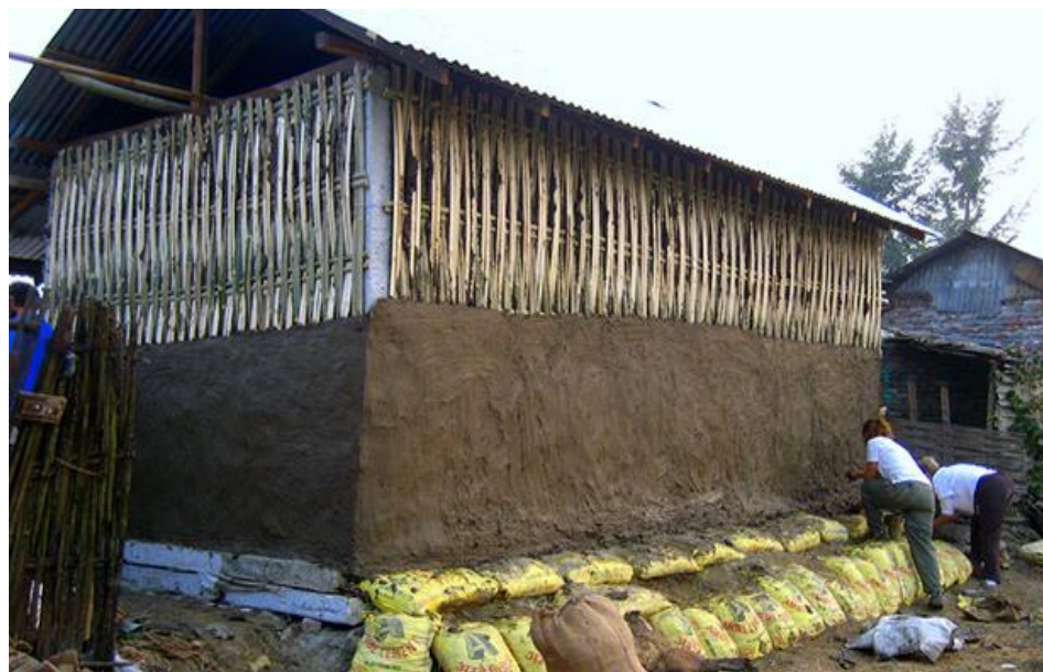
Figure 2.2: Plastering a bamboo-framed house with a cow dug out
