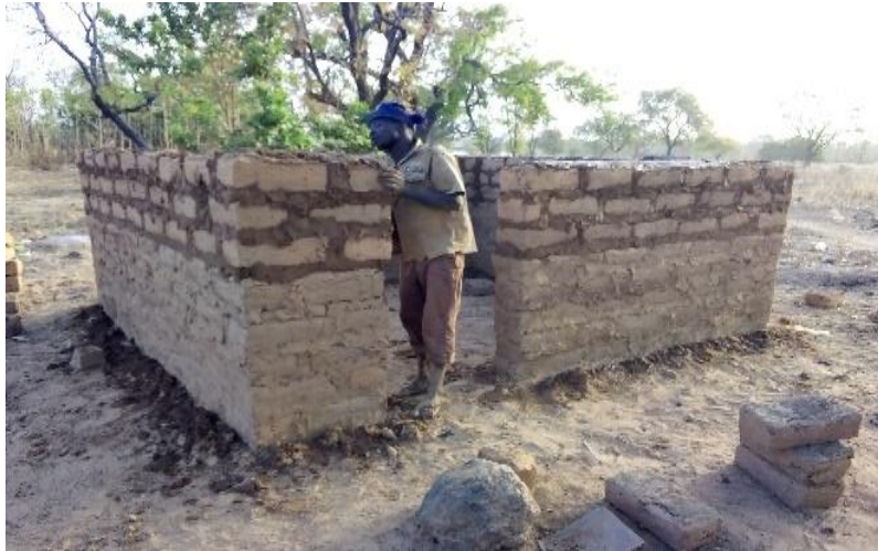
Figure 2.3: A Building Made of Mould Earth Blocks (Source: Charia, Wa Municipal in The Upper West Region)
