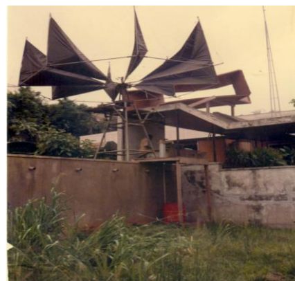
b. Constructed windmill
