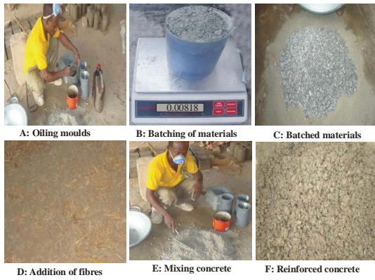
Plate B 3a Preparation of reinforced concrete
